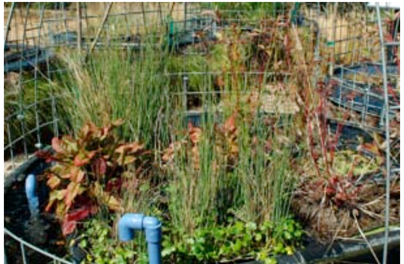
Above and to the left are small-scale plant treatment systems for graywater. The treatment tanks have 'living walls' - which are irrigated by the graywater. This system was built by Paul Kay for demonstration purposes at the Oregon Garden in Silverton.
