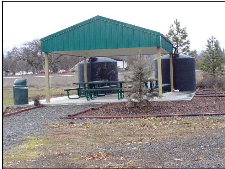
Sam's Valley Elementary School—rainwater catchment system
