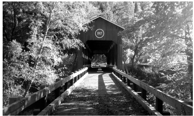
Historic McKee Bridge, Applegate River Valley – built in 1917 by Jason Hartman of Jacksonville.
