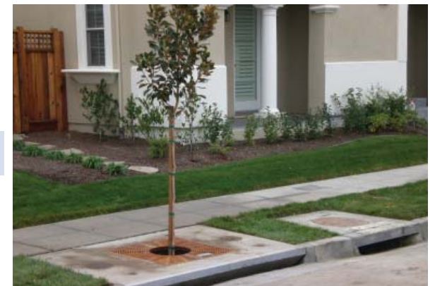
Example of Stormwater Management with Filterra
